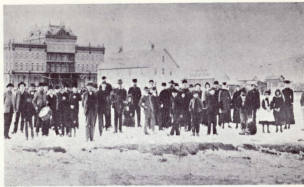
Skating rink east and south of La Veta Hotel provided fun for young and old in 1882. The unfinished La Veta Hotel dominates the background and dwarfs the nearer Edgerton House, which is still standing and is the home of old-timer Roger Teachout. Photo courtesy of Dr. Lois Borland.
