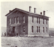
Gunnison County Courthouse in 1881 formed the nucleus for the present building which consists of this section and a number of wings added at various periods of growth, the most recent in 1958-59. Photo courtesy Denver Public Library Western Collection.
