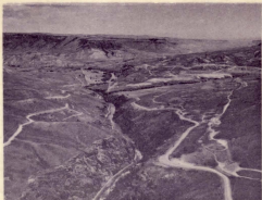
Site of Blue Mesa Dam in the Black Canyon near Sapinero. Photo courtesy U. S. Bureau of Reclamation, Curecanti Unit.
