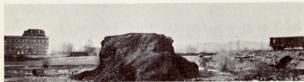
All that remains of the Tomichi Valley Smelter is this huge clinker, dubbed "tar rock" by the younger generation of recent years. The boys found masses of tar clinging to the rock, and pulled off chunks to chew with great gusto. Photo by C. E. Hagie, courtesy Library, State Historical Society of Colorado.
